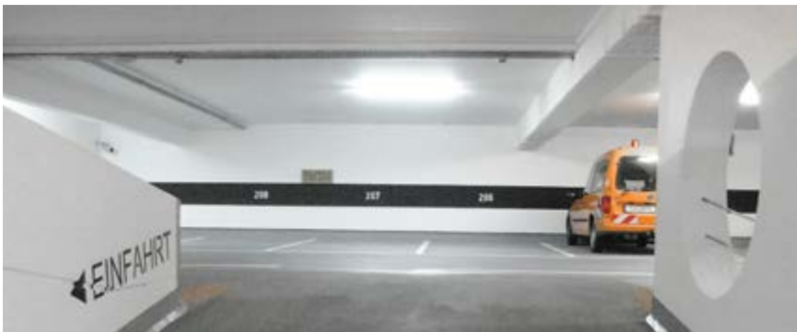
Multi-storey car park West, Überlingen, GER
